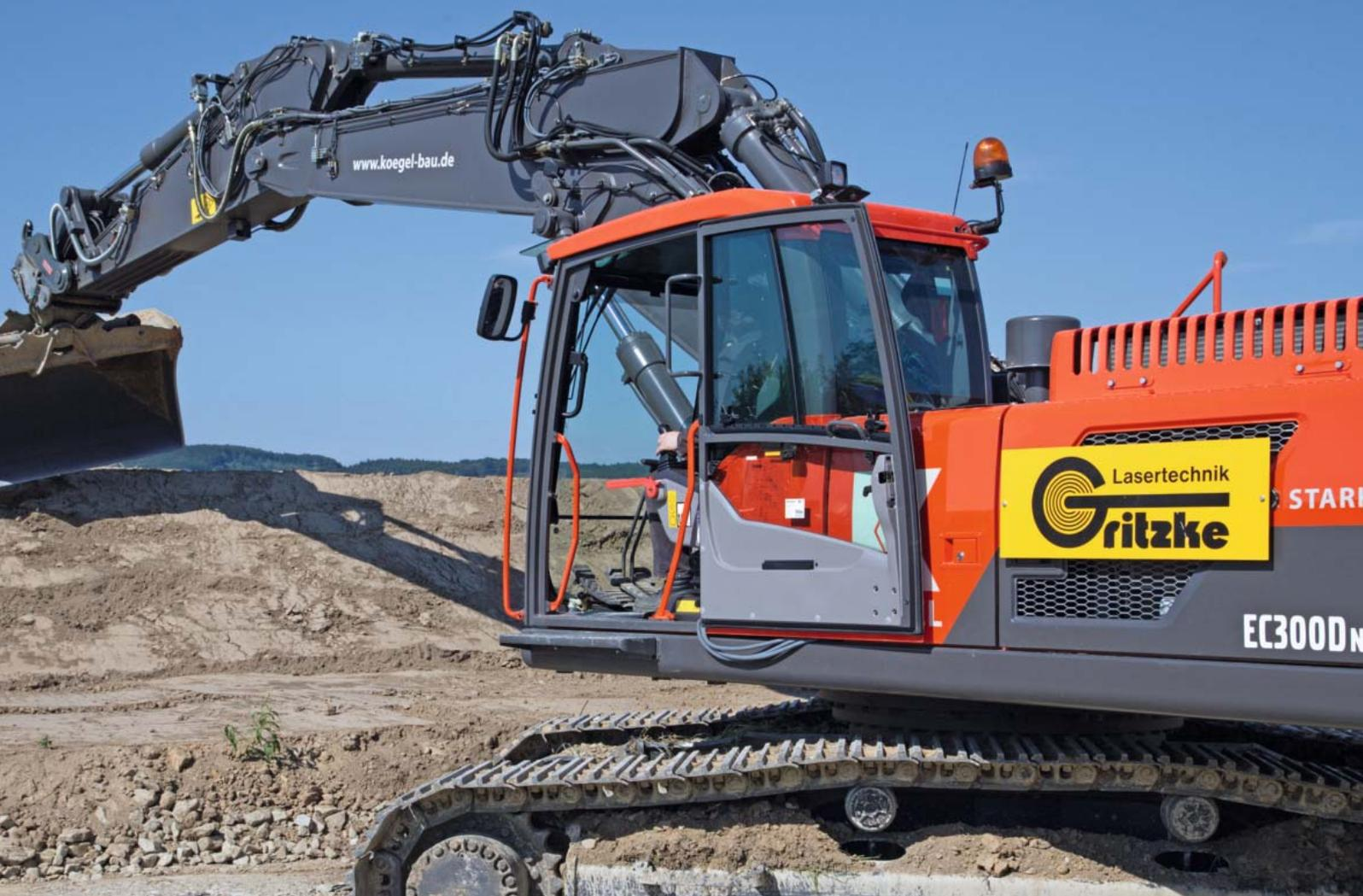
First of all the reference height is levelled by means of the rotation laser and the laser receiver on the adjustable boom of the excavator. Then the planned heights can be determined at any position of the earthworks.
