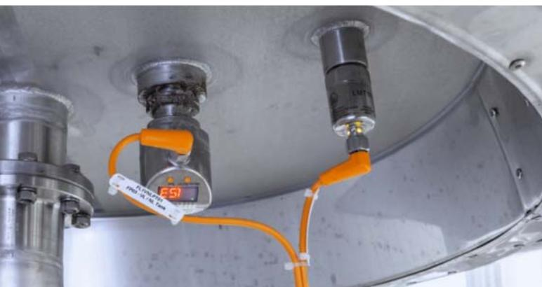
Typical tank monitoring: LMT point level sensor and hydrostatically measuring PI pressure sensor on the tank bottom.
